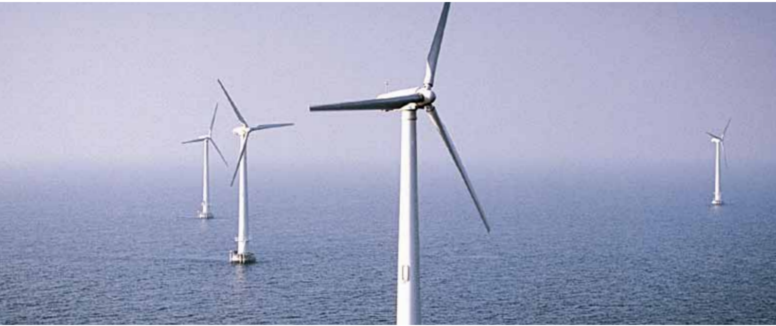
The world's first wind farm at Vindeby, Denmark. Installed by Siemens in 1991. The turbines in this project are still running today
